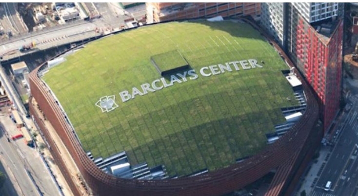
Figure 7: Example of a green roof (Barclays Center, Brooklyn, NY) Source: Weston Solutions
