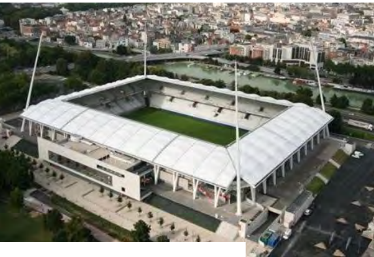
Stade de Reims, whose roof design allows light to reach the pitch
