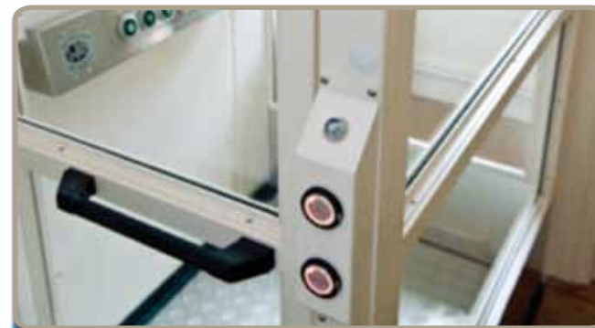
Figure 13 – An enclosed platform lift
