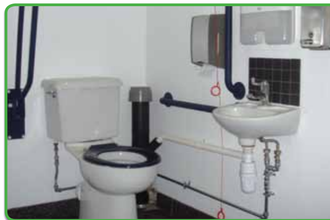
Figure 24 – An example of an accessible toilet
