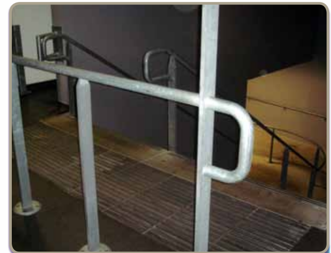
Figure 16 – Tactile paving (detectable warning) with a barrier at the top of the stairs
